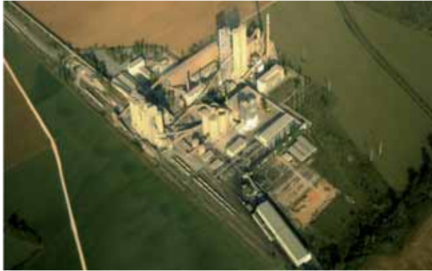
Turna cement plant in Slovakia considerably improved its output and environmental performance thanks to a comprehensive upgrade and expansion programme
