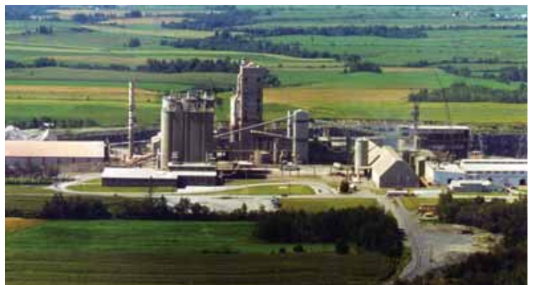
"Cement manufacturing technology" offers students a comprehensive overview of the entire cement production process
